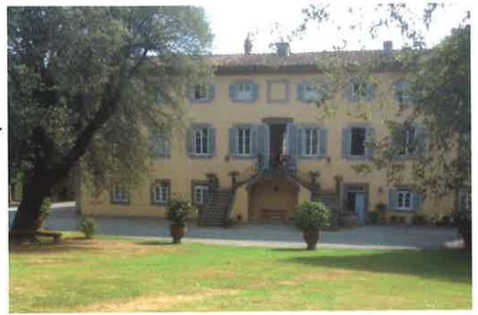
Villa Boccella, Lucca, Italy
